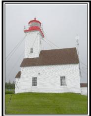
EAST IRONBOUND ISLAND ESTABLISHED: 1867 CCG LIGHT #: 469 44° 26′ 22″ N Position: 64° 05′ 02″ W Near the centre of the island LIGHT: White isophase, F3/E3 AHW: 44.5 metres Nom. RANGE: 12 nautical miles HORN: B3, S27 DESCRIPTION: White rectangular wooden dwelling with tower on one end, 10.8 metres high
