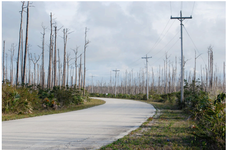
Hurricane damage at Dover Sound
